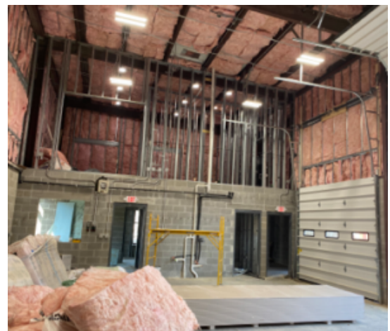
Interior of garage
