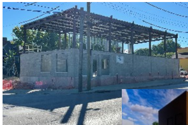
Metal for second story underway
